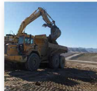
EnergySolutions' Clive disposal facility (Courtesy: EnergySolutions)
