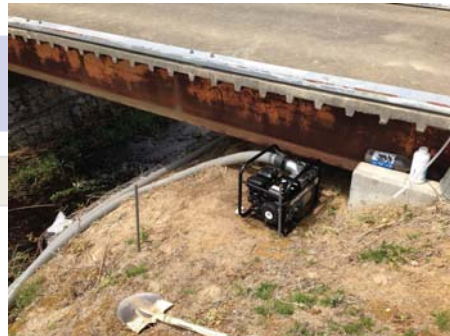
The temporary construction pump
