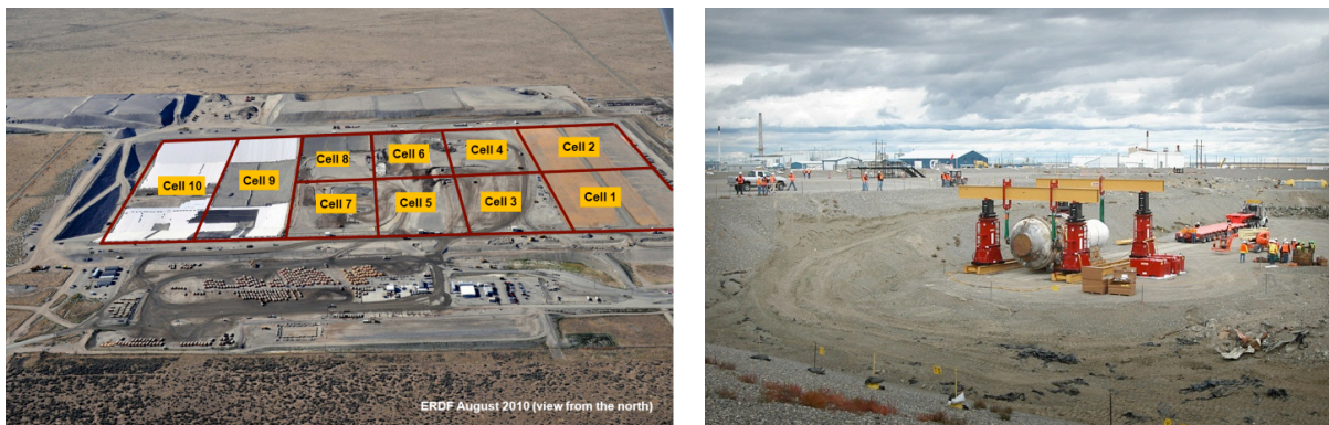
Fig. 1: Facilities with liners and leachate collection systems used for disposal of remediation wastes at the USDOE Hanford (left) and Idaho (right) sites, respectively. The Idaho facility has been used for disposal of reactor vessels from decommissioned test facilities on site as well as a variety of other remediation wastes. (Courtesy: USDOE)
